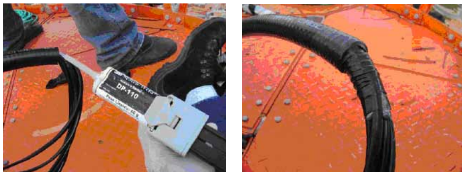
Figure 5: Field termination of hybrid cables.
